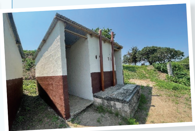
Refurbished learner toilets.
