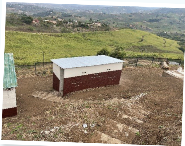
Refurbished learner toilets.
